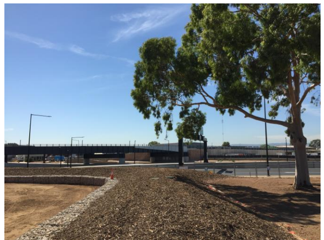
Princes Street basin looking south towards Port Road, March 2019
