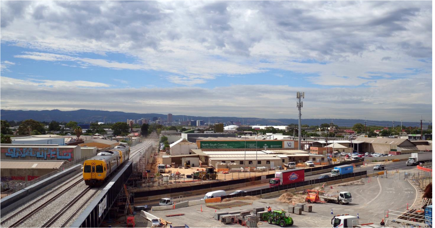
First train service on the Outer Harbor rail overpass - 24 January 2017
